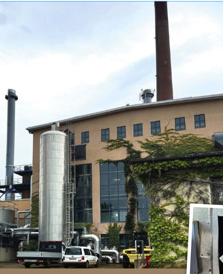
Left: Incineration is a widely adopted method for dealing with materials such as municipal waste, sewage sludge, clinical and hazardous waste, and animal by-products. Pictured is an incinerator in Germany (Picture credit: Signal Group)
